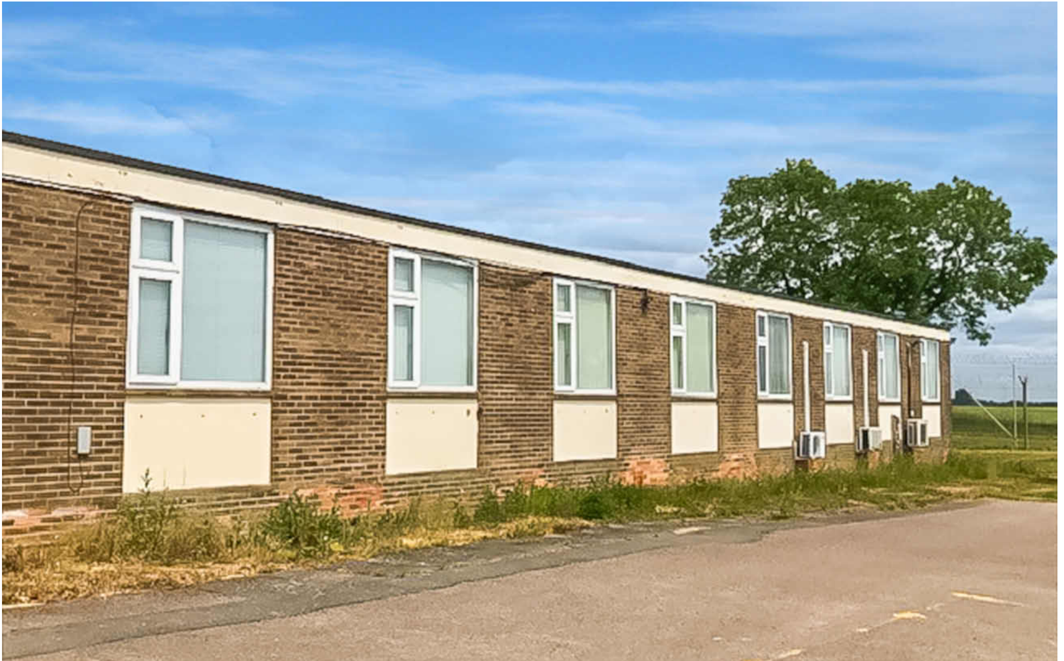
Office 1 & Store 1a, Signals House, Bampton Business Centre North, TO LET - £3,150 p.a.x.
