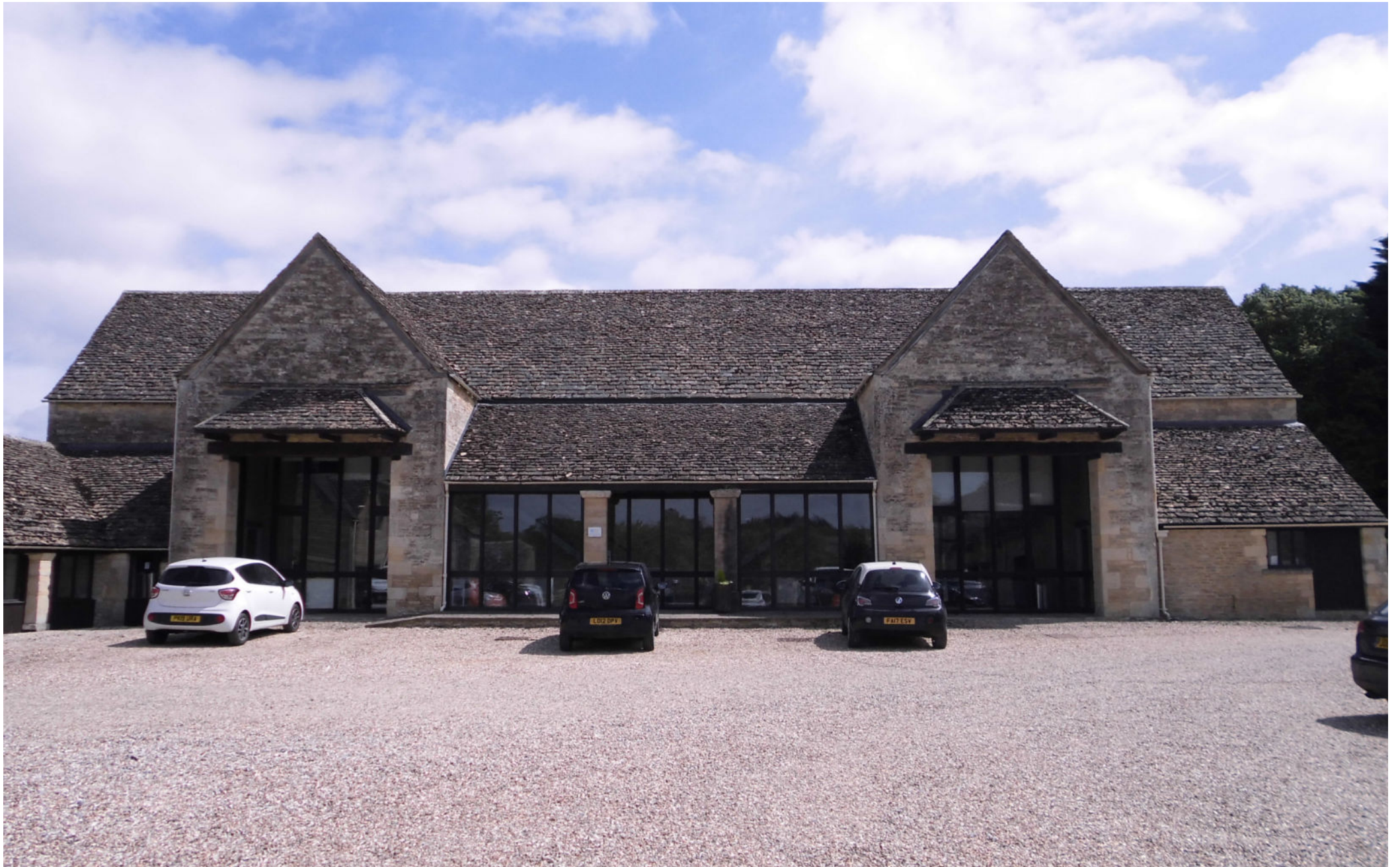
Unit 2 & Unit 3, Tithe Barn, Barnsley Park Estate,
