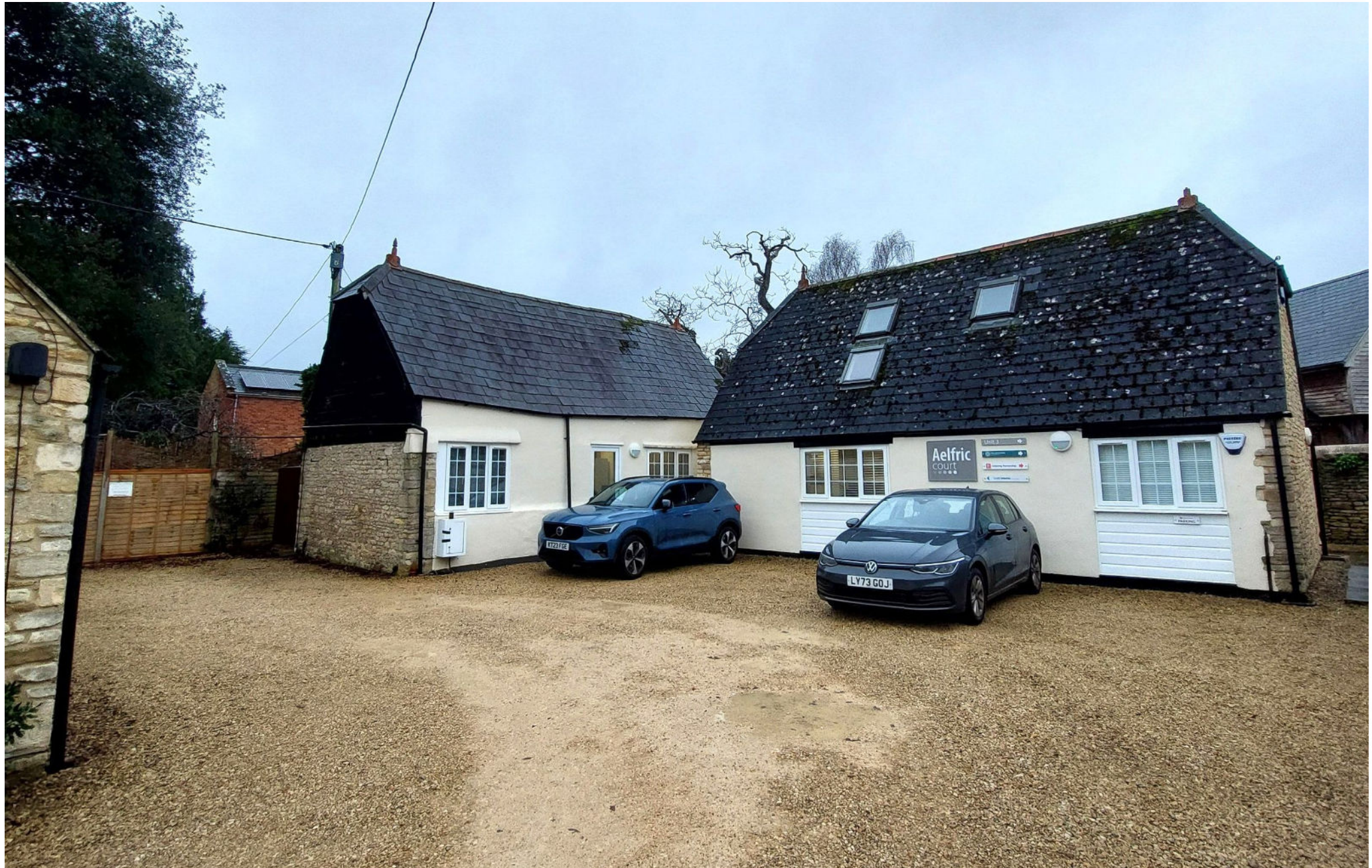
Aelfric Court, 2 Oxford Road, Eynsham, Oxfordshire
