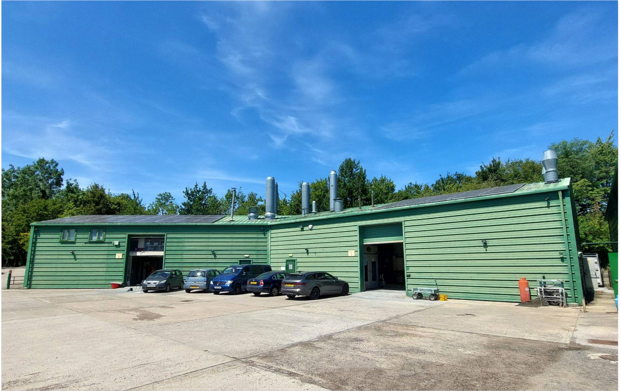
Unit 4 and Unit 5, Brick Kiln Works, Childrey, Wantage, Oxon TO LET - £45,000 p.a.x.
